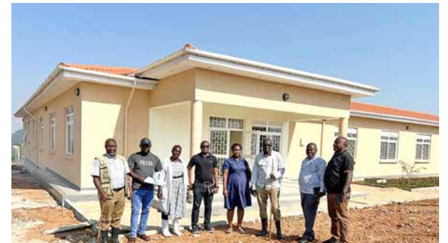
Buyana Students Hostel nearing completion
